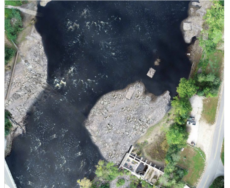
Photo 11-3 Post-Full Spillway Removal Aerial View of Bar Mills Dam
