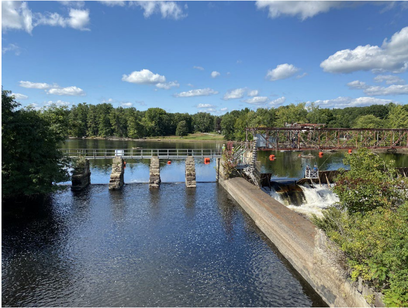
Photo 11-10 Existing View of Bar Mills Dam from Canal
