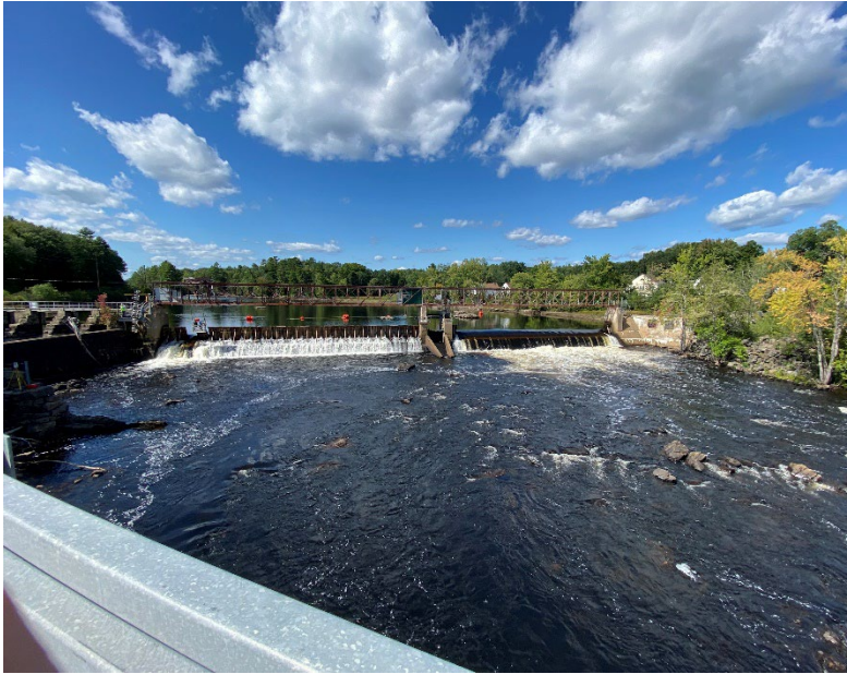
Photo 11-4 Existing View of Bar Mills Dam from Bar Mills Bridge
