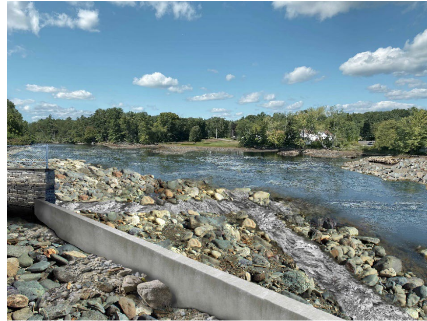
Photo 11-11 Post-Breach and Full Spillway Removal View of Bar Mills Dam from Canal
