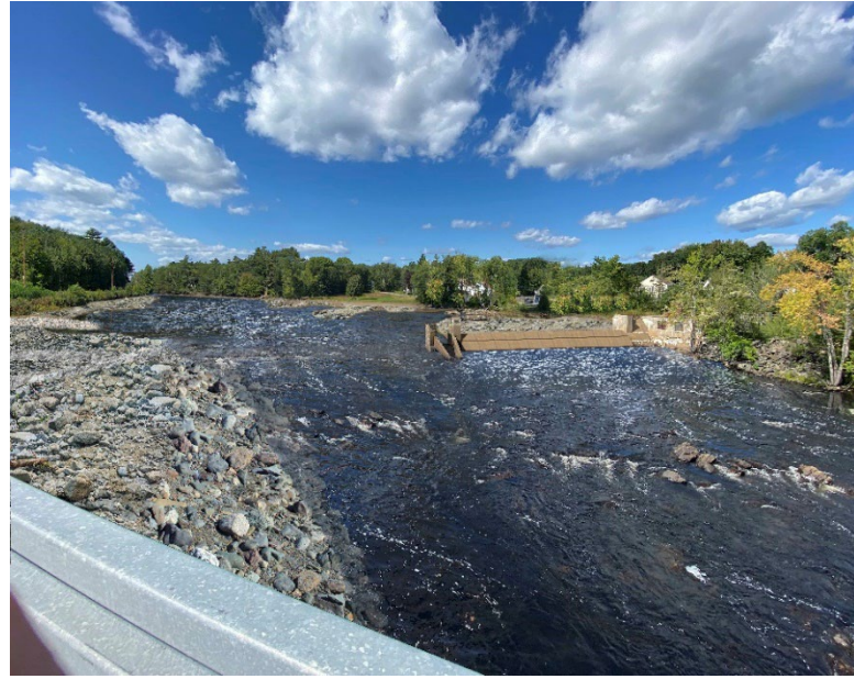
Photo 11-5 Post-Partial Breach View of Bar Mills Dam from Bar Mills Bridge
