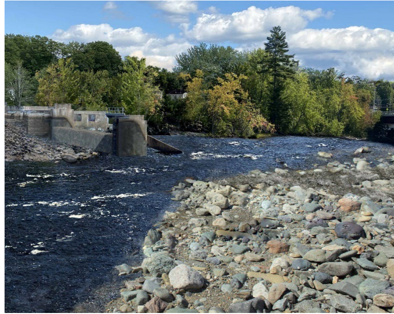
Photo 11-8 Post-Partial Breach View of Bar Mills Dam from Boat Launch
