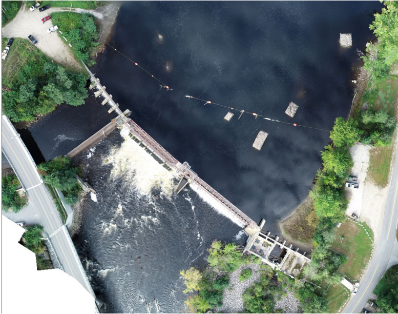
Photo 11-1 Existing Aerial View of Bar Mills Dam
