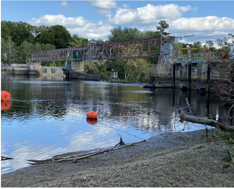
Photo 11-7 Existing View of Bar Mills Dam from Boat Launch
