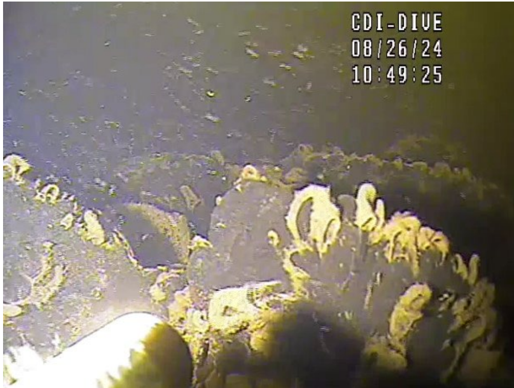
Photo 5-3 Underwater Imagery Immediately Upstream of Bar Mills Dam
