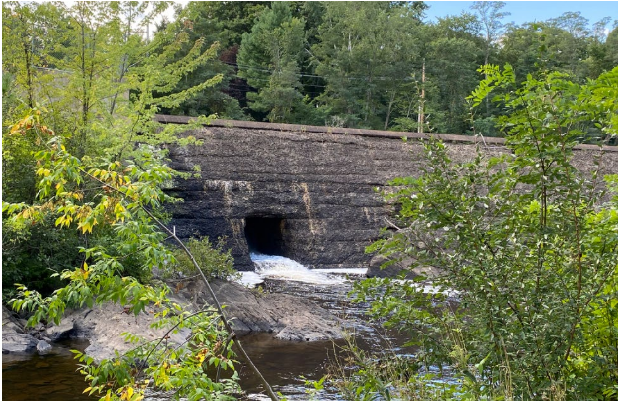
Photo 1-5 Downstream Side of Powerhouse Spillway and Canal Drain Gate
