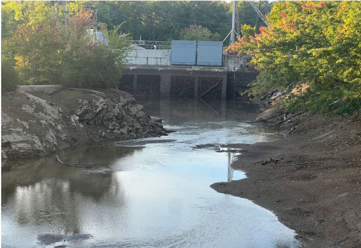
Photo 1-4 Canal Looking from Bridge Towards Powerhouse Under Drawdown
