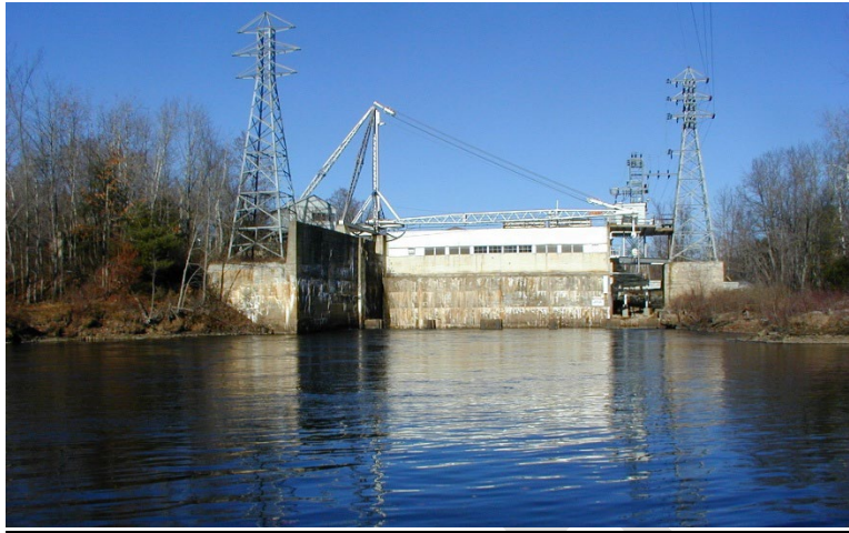
Photo 1-7 View of Powerhouse from Downstream
