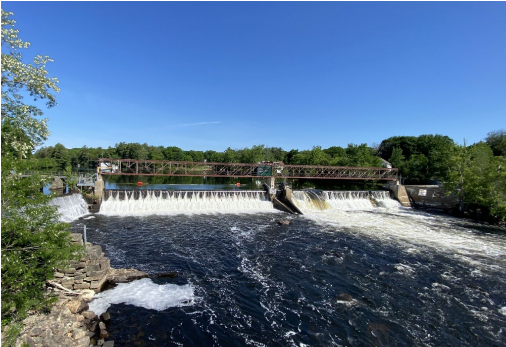
Photo 3-1 Downstream View of Spillway
