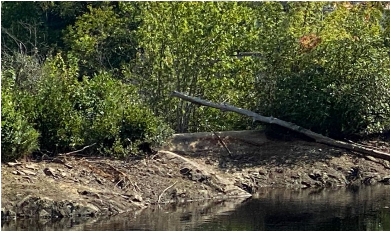
Photo 2-1 Typical Saddle Dam in Canal to Remain
