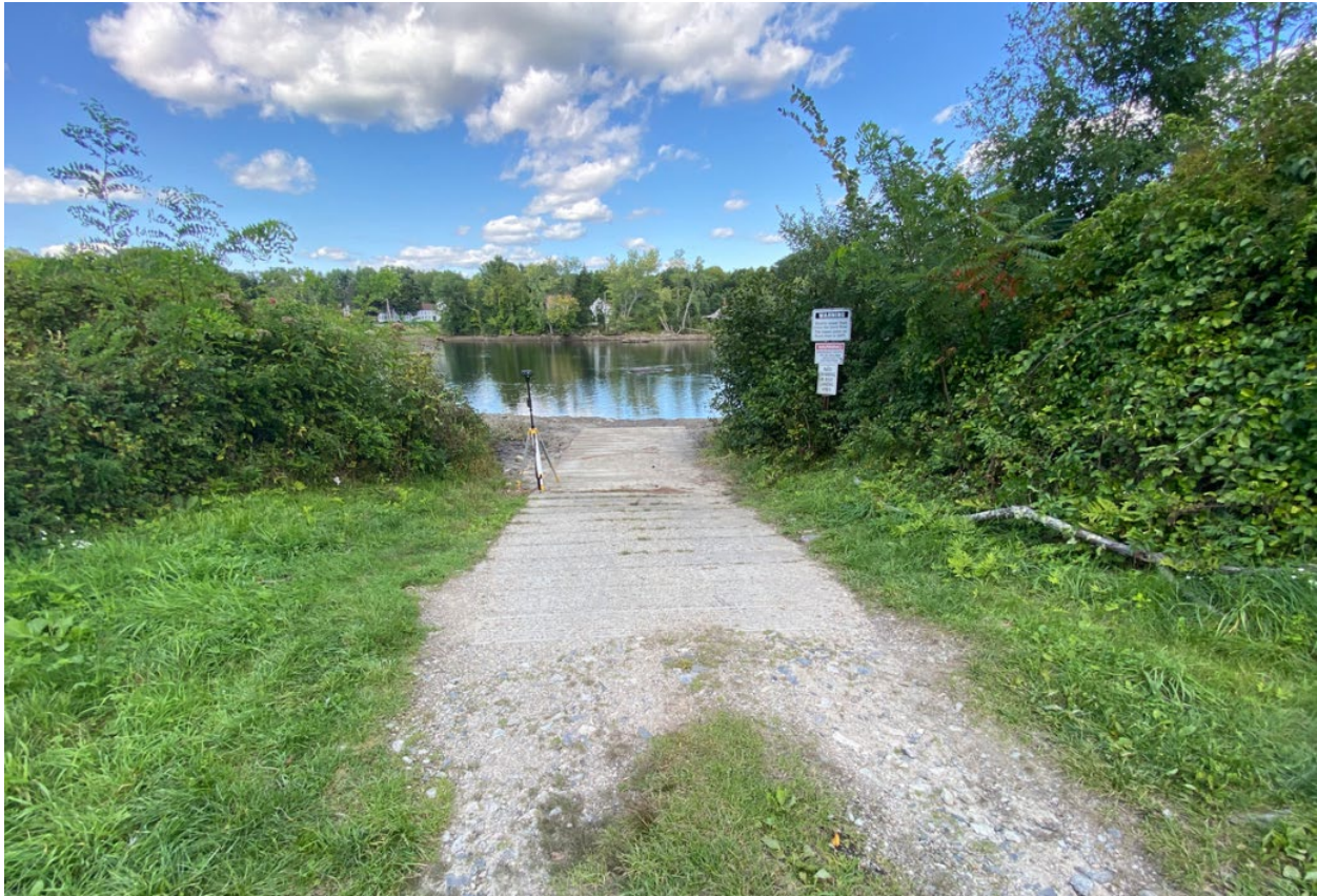
Photo 2-3 Existing Boat Launch
