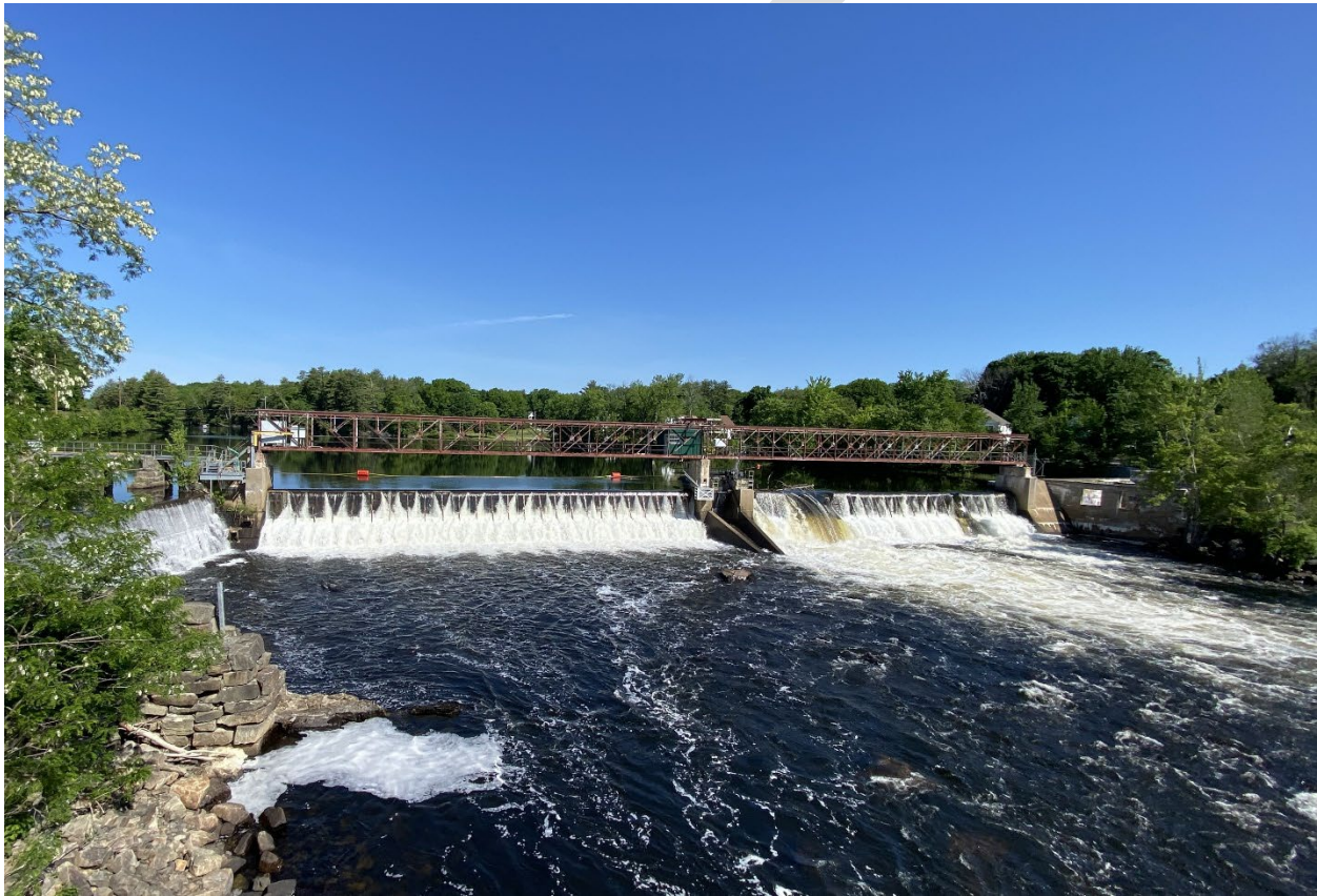
Photo 1-1 Downstream View of Spillway
