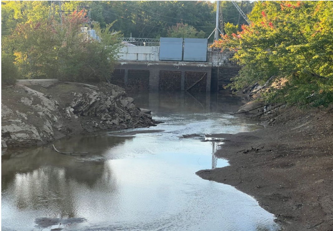
Photo 3-3 Canal Looking from Bridge Towards Powerhouse Under Drawdown
